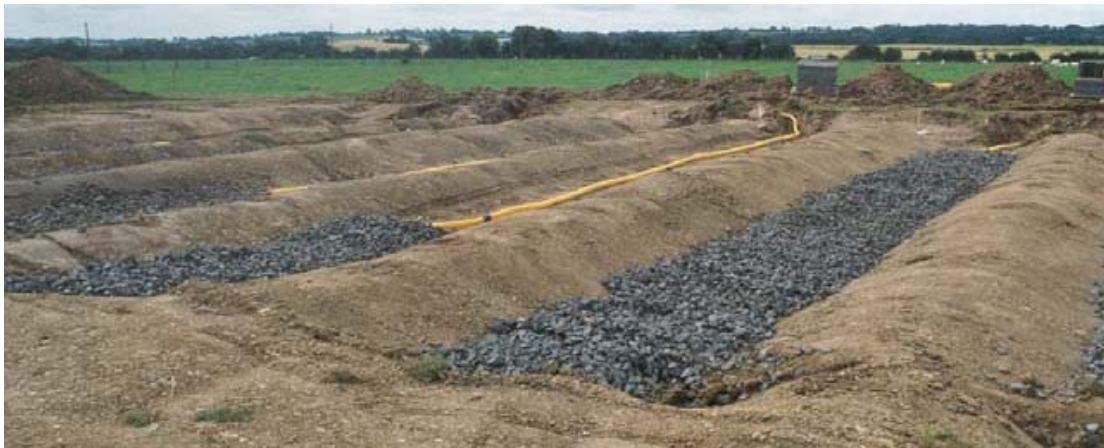
Figure A2. Compacted subsoil ridges in a subsoil-lined OWP effluent collection system.
